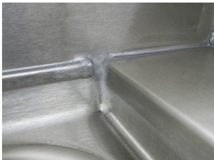
Soldered and Siliconed Seams
